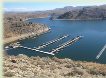
Marina Dock Replacement
