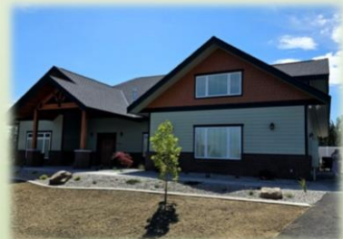
Design-Build New Construction
