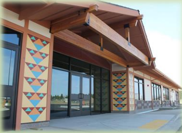
10,000sf New Construction
