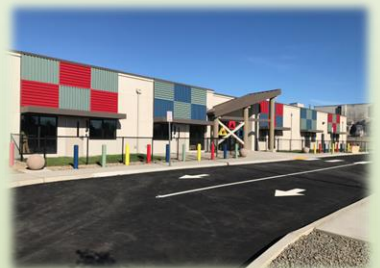
17,000sf New Construction
