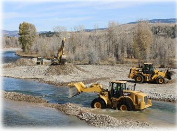
Road & Bank Stabilization
