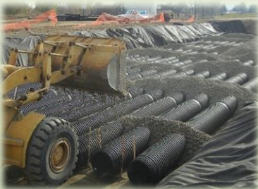
Parking Lot & Infiltration Gallery
