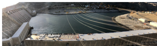
$7.8M Grand Coulee 3rd Powerplant Roof Replacement, BOR
