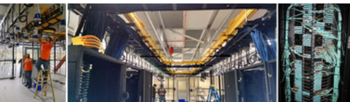
$1.3M Western Processing Center (WPC) Relocation, ACE-IT
