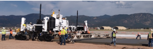
$14.5M Alpha Ramp Repair, USACE Ft. Carson
