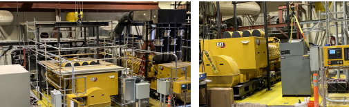
$12M Replace Generators, Schriever Space Force
