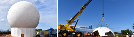
$1.3M RASP Antenna Installation Wahiawa, ATC
