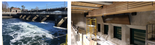
$767K Fish Ladder Working Area Remodel, LWSC
